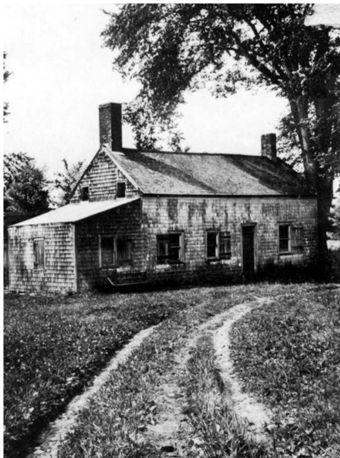
Caretaker's Cottage at Rookwood, Fredericton, N.B.
