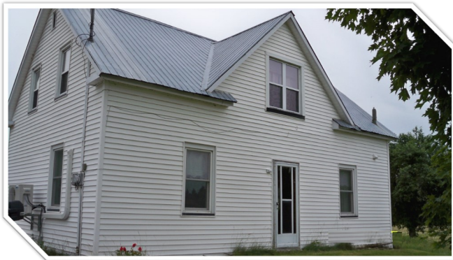
The KING homestead in Douglasfield
